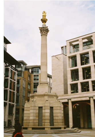
“Cunningly disguised ventilation shaft”
